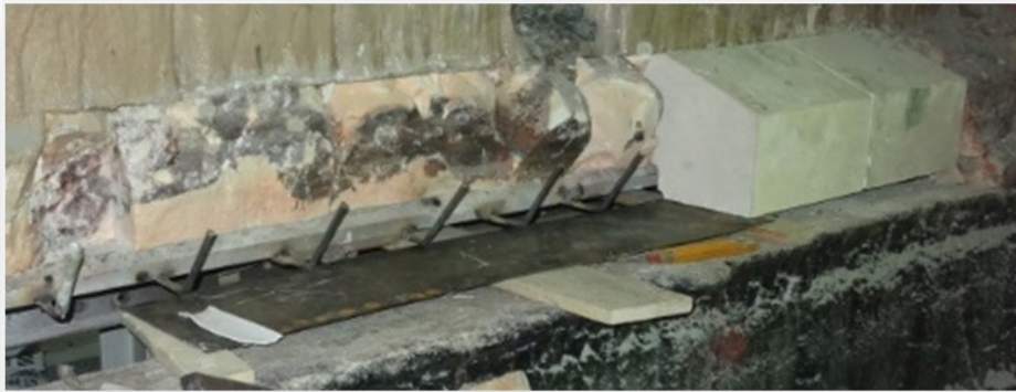
Tuckstones - Partial Cold Repair
