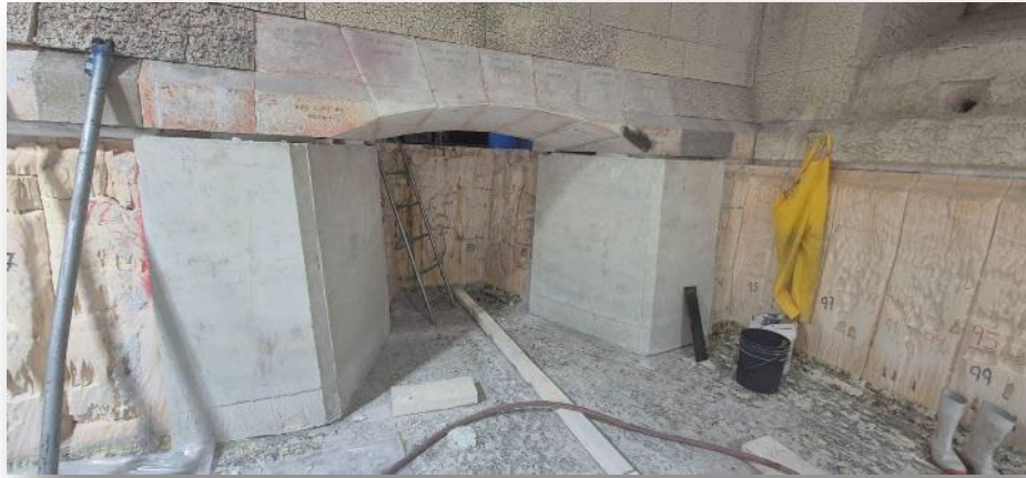
Sidewall or Dog House - Partial or Major Cold Repair
